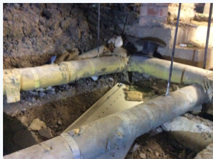
ITEM NO.: 1 PHOTO NO.: J161155-03-ISLHD-PKH-E-PHOTO042 RESULT: SMF - PRESUMED POSITIVE BUILDING/LEVEL: STAFF QUARTERS, OLU & INTERPRETERS - SUB FLOOR ROOM/LOCATION: SUB FLOOR - NORTHEAST FEATURE/MATERIAL: PIPEWORK INSULATION - INSULATION MATERIAL SAMPLE NO.: -
