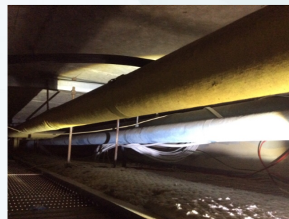
ITEM NO.: 20 PHOTO NO.: J161155-03-ISLHD-PKH-E-PHOTO010 RESULT: SMF - PRESUMED POSITIVE BUILDING/LEVEL: STAFF QUARTERS, OLU & INTERPRETERS - LEVEL 01 ROOM/LOCATION: CORRIDOR PKBE0191 - THROUGHOUT FEATURE/MATERIAL: PIPEWORK INSULATION - INSULATION MATERIAL SAMPLE NO.: -
