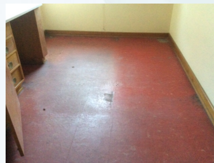
ITEM NO.: 34 PHOTO NO.: J161155-03-ISLHD-PKH-E-PHOTO026 RESULT: ASBESTOS - PREVIOUSLY SAMPLED NEGATIVE BUILDING/LEVEL: STAFF QUARTERS, OLU & INTERPRETERS - LEVEL 02 ROOM/LOCATION: VARIOUS ROOMS - THROUGHOUT FEATURE/MATERIAL: FLOOR COVERING - VINYL TILES SAMPLE NO.: PREVIOUSLY SAMPLED GREENCAP J149255-03-PKDH - E-007
