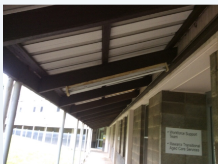
ITEM NO.: 5 PHOTO NO.: J161155-03-ISLHD-PKH-E-PHOTO001 RESULT: PCB - PRESUMED POSITIVE BUILDING/LEVEL: STAFF QUARTERS, OLU & INTERPRETERS - LEVEL 00 ROOM/LOCATION: VERANDAH - WEST FEATURE/MATERIAL: FLUORESCENT LIGHT FITTING - CAPACITOR SAMPLE NO.: -
