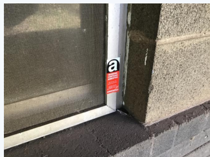
ITEM NO.: 17 PHOTO NO.: J161155-03-ISLHD-PKH-E-PHOTO053 RESULT: ASBESTOS - PREVIOUSLY SAMPLED POSITIVE BUILDING/LEVEL: STAFF QUARTERS, OLU & INTERPRETERS - LEVEL 01 ROOM/LOCATION: - SURROUNDING FEATURE/MATERIAL: WINDOW FRAMES - PUTTY SAMPLE NO.: PREVIOUSLY SAMPLED GREENCAP J149255-03-PKDH - E-003
