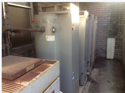
ITEM NO.: 3 PHOTO NO.: J161155-03-ISLHD-PKH-E-PHOTO039 RESULT: SMF - PRESUMED POSITIVE BUILDING/LEVEL: STAFF QUARTERS, OLU & INTERPRETERS - LEVEL 00 ROOM/LOCATION: - SOUTHEAST FEATURE/MATERIAL: HOT WATER HEATER - INSULATION MATERIAL SAMPLE NO.: -
