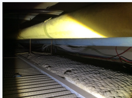
ITEM NO.: 19 PHOTO NO.: J161155-03-ISLHD-PKH-E-PHOTO011 RESULT: SMF - PRESUMED POSITIVE BUILDING/LEVEL: STAFF QUARTERS, OLU & INTERPRETERS - LEVEL 01 ROOM/LOCATION: CORRIDOR PKBE0191 - THROUGHOUT FEATURE/MATERIAL: INSULATION - INSULATION BATTS SAMPLE NO.: -
