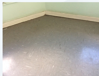
ITEM NO.: 36 PHOTO NO.: J161155-03-ISLHD-PKH-E-PHOTO029 RESULT: ASBESTOS - PREVIOUSLY SAMPLED NEGATIVE BUILDING/LEVEL: STAFF QUARTERS, OLU & INTERPRETERS - LEVEL 02 ROOM/LOCATION: VARIOUS ROOMS - THROUGHOUT FEATURE/MATERIAL: FLOOR COVERING - VINYL TILES SAMPLE NO.: PREVIOUSLY SAMPLED GREENCAP J149255-03-PKDH - E-010
