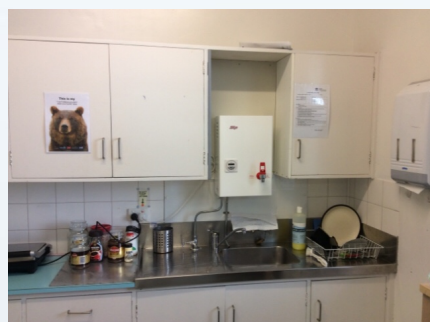
ITEM NO.: 21 PHOTO NO.: J161155-03-ISLHD-PKH-E-PHOTO005 RESULT: SMF - PRESUMED POSITIVE BUILDING/LEVEL: STAFF QUARTERS, OLU & INTERPRETERS - LEVEL 01 ROOM/LOCATION: KITCHEN PKBE0110 - EAST FEATURE/MATERIAL: HOT WATER HEATER - INSULATION MATERIAL SAMPLE NO.: -
