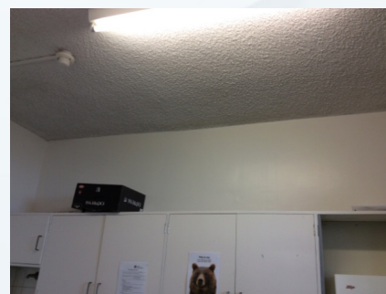
ITEM NO.: 22 PHOTO NO.: J161155-03-ISLHD-PKH-E-PHOTO006 RESULT: ASBESTOS - PRESUMED NEGATIVE BUILDING/LEVEL: STAFF QUARTERS, OLU & INTERPRETERS - LEVEL 01 ROOM/LOCATION: KITCHEN PKBE0110 - THROUGHOUT FEATURE/MATERIAL: CEILING - SPRAYED VERMICULITE SAMPLE NO.: PREVIOUSLY SAMPLED GREENCAP SIMILAR TO J149255-03-PKDH - E-002
