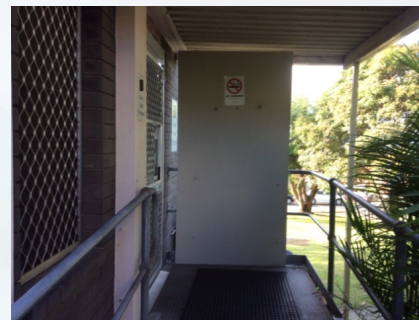
ITEM NO.: 2 PHOTO NO.: J161155-03-ISLHD-PKH-E-PHOTO038 RESULT: ASBESTOS - PREVIOUSLY SAMPLED NEGATIVE BUILDING/LEVEL: STAFF QUARTERS, OLU & INTERPRETERS - LEVEL 00 ROOM/LOCATION: - SOUTH FEATURE/MATERIAL: WALL CLADDING - COMPRESSED CEMENT SHEETING SAMPLE NO.: PREVIOUSLY SAMPLED GREENCAP J149255-03-PKDH - E-011
