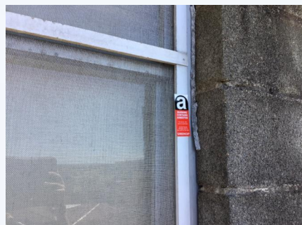
ITEM NO.: 33 PHOTO NO.: J161155-03-ISLHD-PKH-E-PHOTO055 RESULT: ASBESTOS - PRESUMED POSITIVE BUILDING/LEVEL: STAFF QUARTERS, OLU & INTERPRETERS - LEVEL 02 ROOM/LOCATION: LOUNGE PKBE0225 - SURROUNDING FEATURE/MATERIAL: WINDOW FRAMES - PUTTY SAMPLE NO.: PREVIOUSLY SAMPLED GREENCAP SIMILAR TO J149255-03-PKDH - E-003
